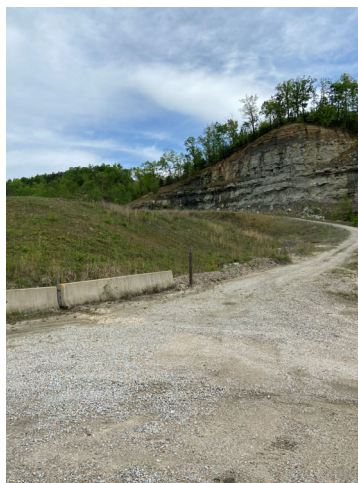
Figure 7. Artificial fill from mine activities.
